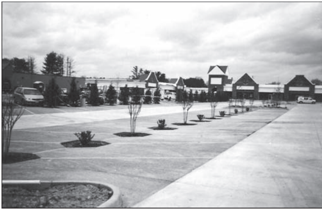
Figure 12. Parking for prime outlets mall in Williamsburg, Virginia (7.6 acres)
