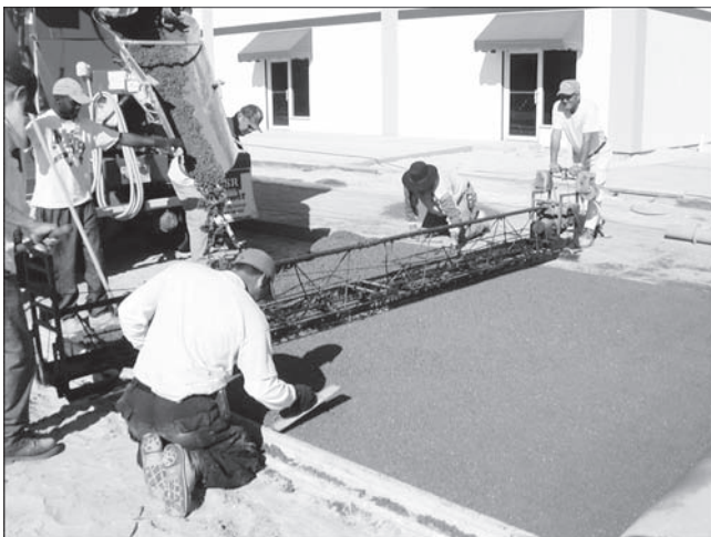
Figure 8. Pervious concrete struck off by vibratory screed
