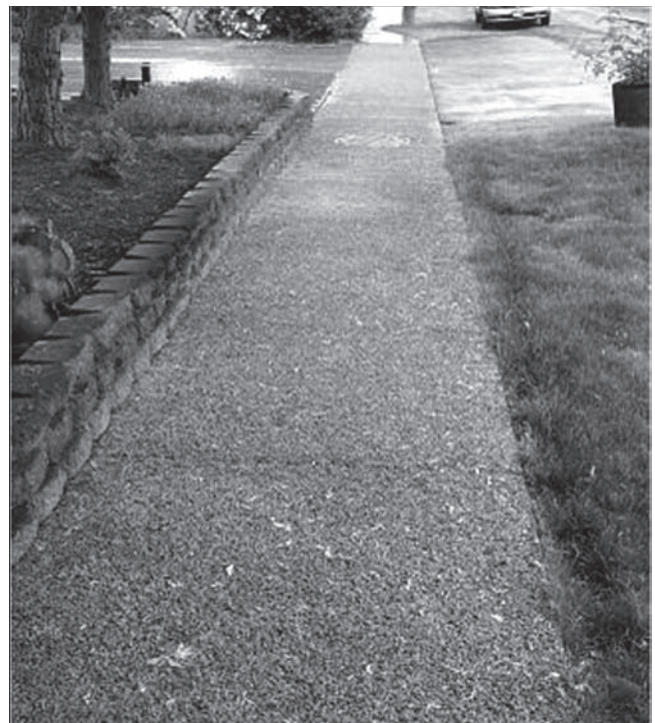
Figure 3c. Pervious concrete application - Sidewalks
