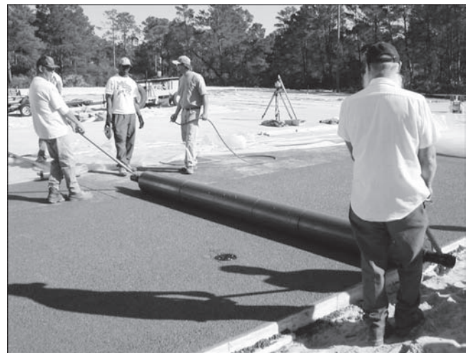
Figure 9. Example of compaction of pervious concrete by rolling
