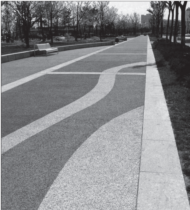
Figure 13. Walkway in Beijing, China built for 2008 Olympics
