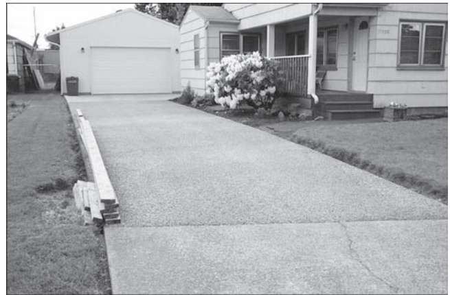
Figure 3b. Pervious concrete application - Driveways
