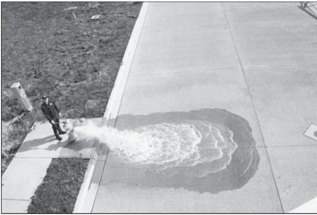
Figure 2. Pervious concrete residential street showing water infiltration
